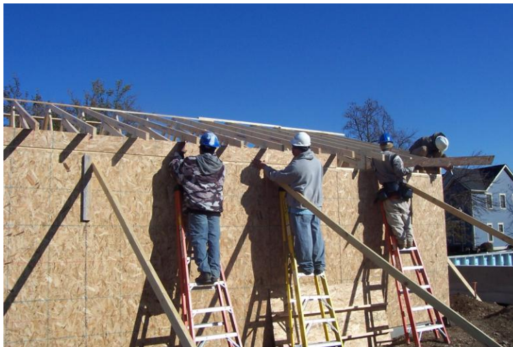
ISUS, Hands-on Construction Training
